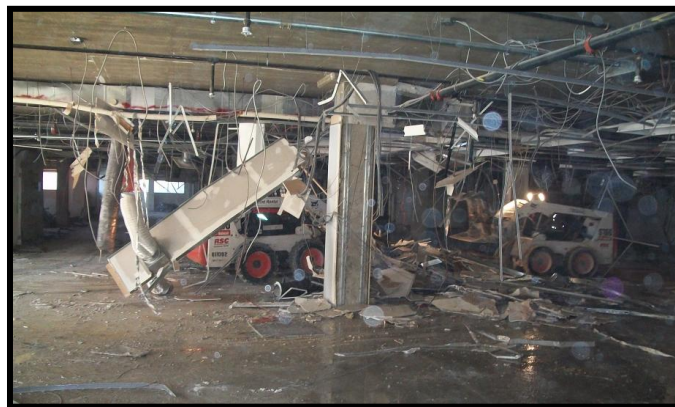
Figure 4: Ceiling Demolition at 7700 Arlington Blvd.
